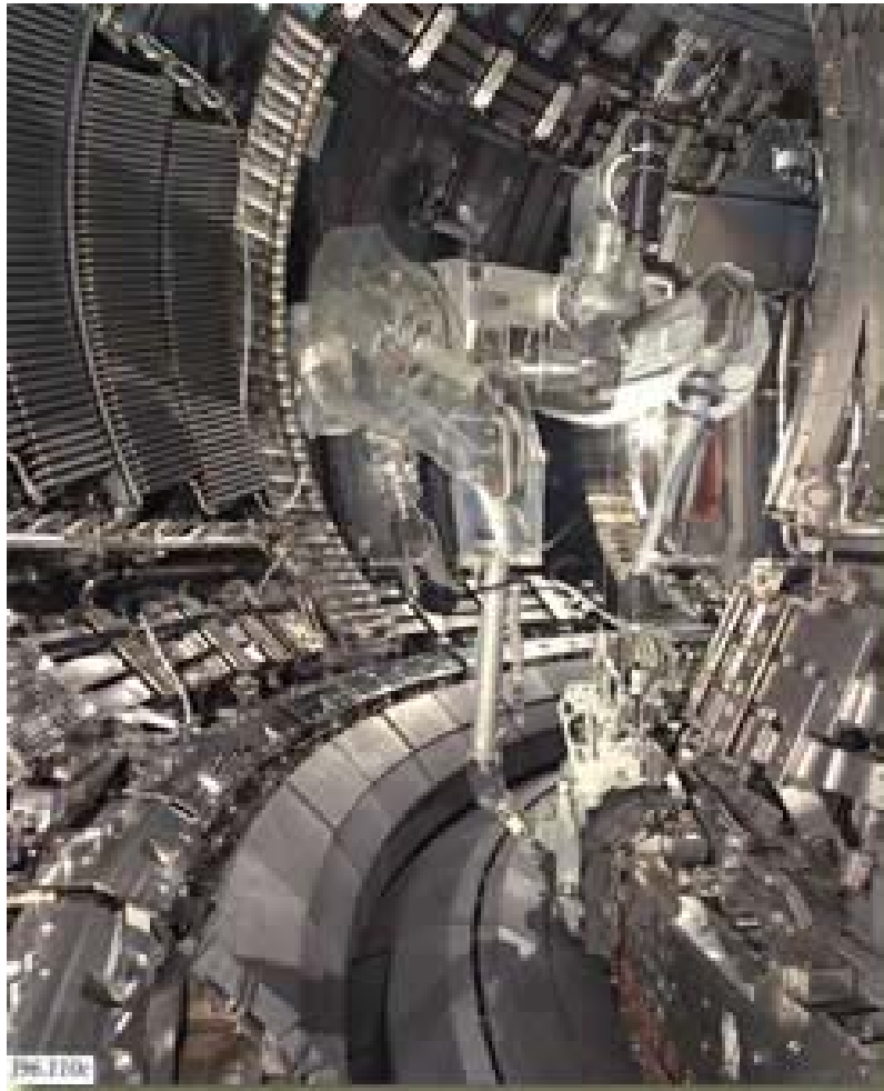
Figure 5 – Manipulator installing the tiles of the JET Mark II divertor
